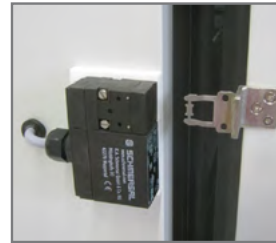
Electromechanical door lock mechanism controlled in a program and/or manually
