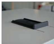
Manually adjustable exhaust air flap
